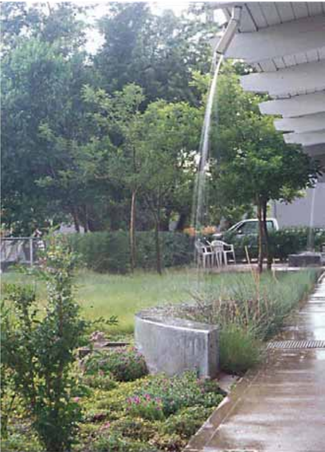
GARDEN SUPPORTED BY ROOF RUNOFF Runoff drains through a spout from the roof to a splash basin behind the curved walls and to a rain garden on the left. Drought tolerant native and non-native plants can withstand wet and dry cycles.
