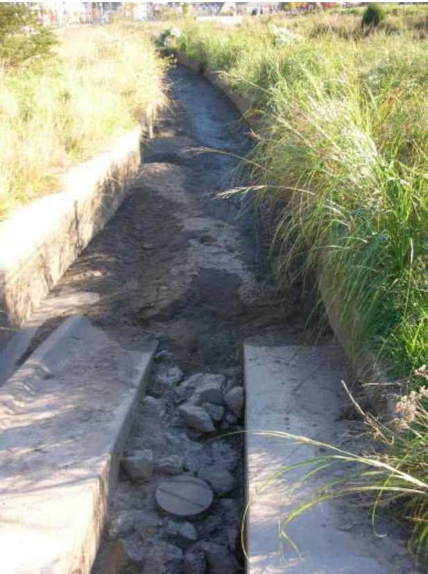
SMALL STORMWATER PIPE SEDIMENT TRAP This sediment basin also functions as a level spreader which disperses flows to the PLD on the right. The ramps, which have a small pipe outfalling between them, extend the length of the trap as concrete tracks allowing access by a Bobcat for sediment removal. Infiltration occurs in pervious soils between the tracks.
