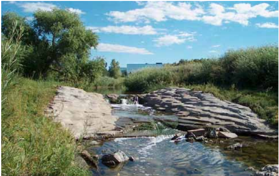
SCULPTED SHOTCRETE CHECK STRUCTURE The small, stepped drops and pools allow movement of fish and macro invertebrates, and allow safe pedestrian water access.
