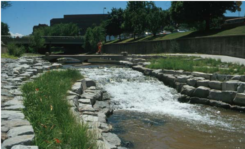
SLOPED GROUTED RIP-RAP DROP STRUCTURE This structure extends from the vertical wall on the right to a wall out of the photo on the left. Plantings are in grouted rip-rap basins. Rip-rap lining of the plunge pool at the base of the structure is buried to diminish the visual mass of the structure. The stepped low flow is a preferred design, allowing movement of fish and macro invertebrates. Terraced side slopes allow safe pedestrian access to the waters edge.
