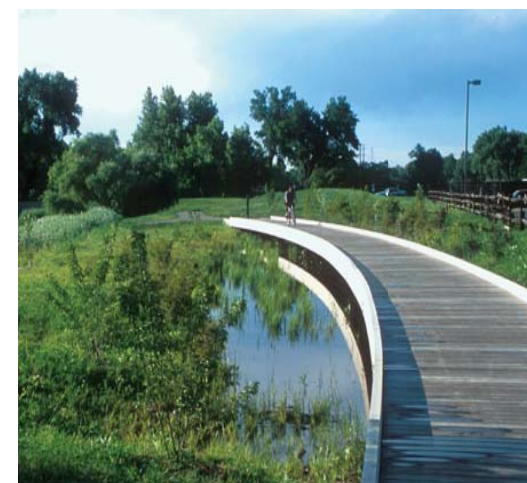
This PLD treats runoff from the parking area to the right of the photo. The small pocket wetland complements the natural qualities of the stream corridor to the left, and provides an enhanced experience for trail users.
