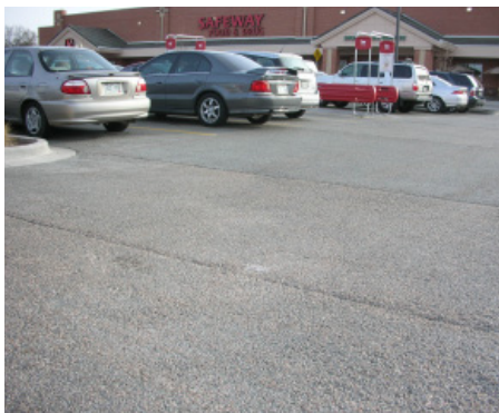
Poured-in-place concrete porous pavement can be substituted for standard asphalt or concrete pavement.
