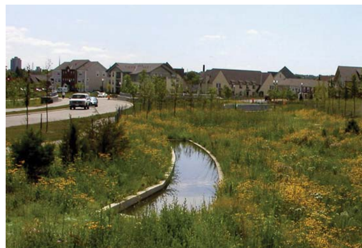
This larger PLD in a medium density neighborhood gives identity to the community. Native mesic prairie shown can tolerate wet and dry periods. The sediment trap shown filled with water following a storm event in this photo, is shown on page 49 in more detail.
