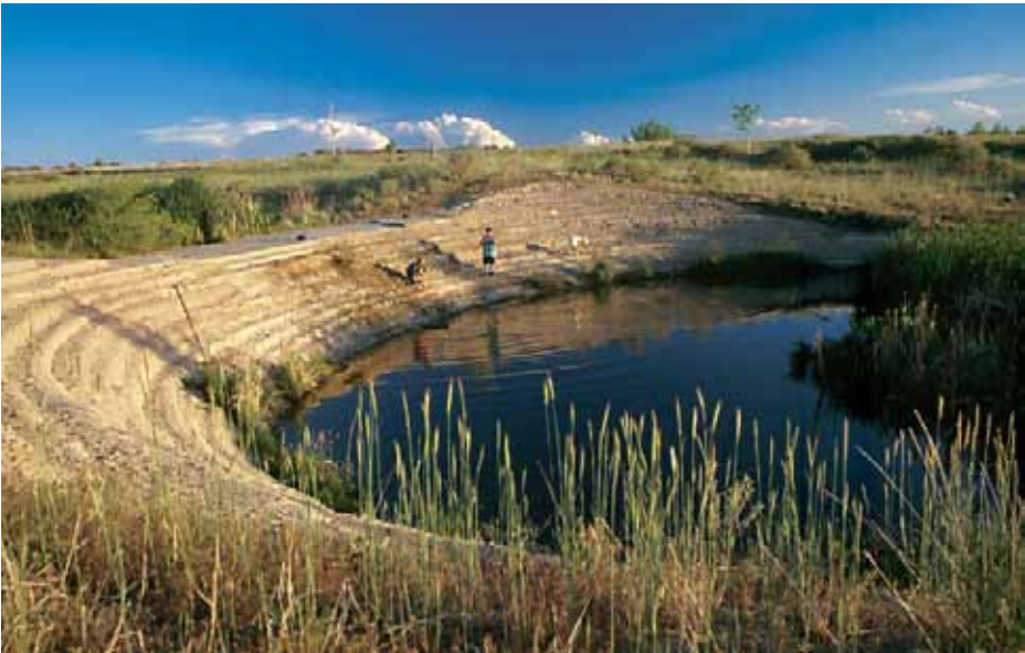
SOIL CEMENT DROP STRUCTURE The structure blends into its natural prairie setting. Small terraces created by the layered installation of soil cement makes it safe. Aquatic habitat value is limited because low flows are piped through the structure.
