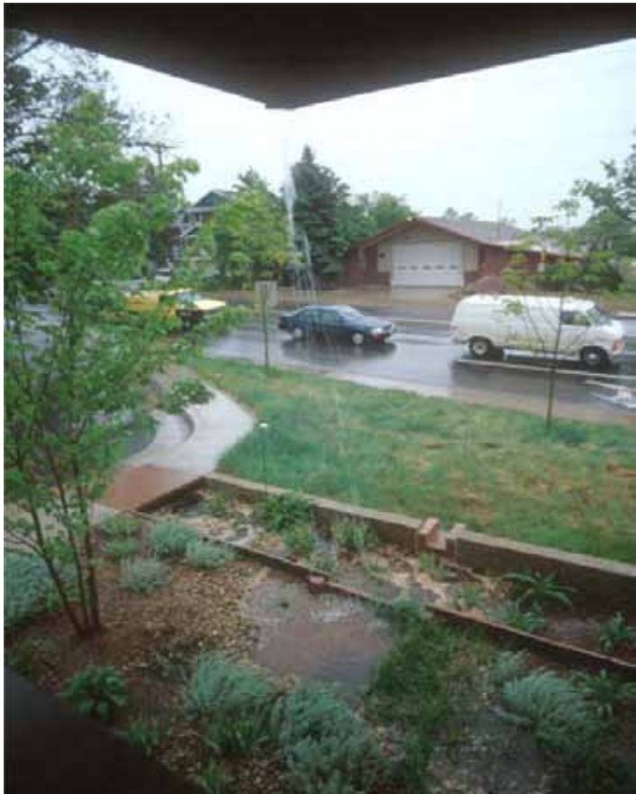
PLANTER GARDEN SUPPORTED BY ROOF RUNOFF Runoff drains to an infiltration planter that is lined to prevent building damage. Overflows drain to adjacent grass swales, plants were selected to accommodate wet and dry cycles.
