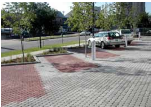
Modular block porous pavement in this small parking lot allows water from the adjacent building, as well as the parking lot itself to infiltrate.
