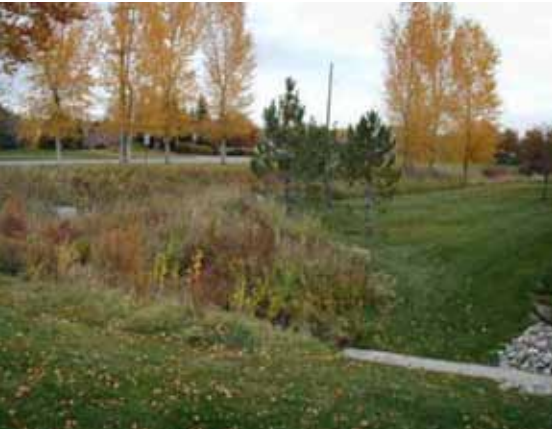
DETENTION BASIN WET MEADOW OR MESIC PRAIRIE Wetland grasses planted in the bottom of this detention basin remove nutrients and pollutants from stormwater runoff, require minimal maintenance, and can be easily replaced if sediments must be removed.
