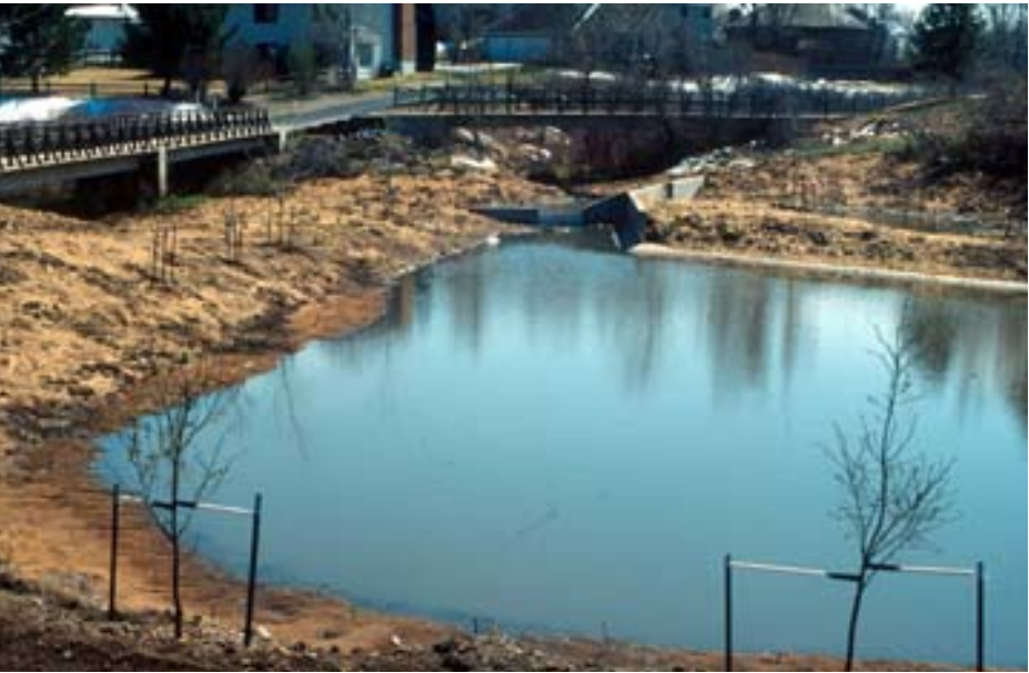
SEDIMENT POND This on-line pond collects large volumes of sediment from a small urbanized watershed. Creek flows can be redirected and the pond can be drained to allow access by large equipment.
