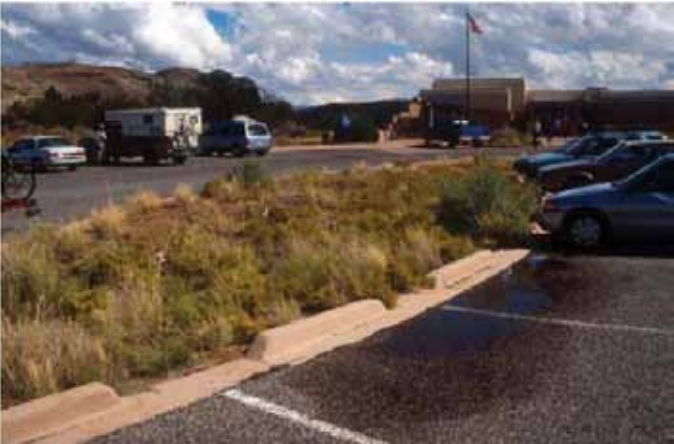
SLOTTED CURB SPREADER The slotted curb in this parking lot area has depressions between each parking space to allow runoff to flow to the interior landscape area without concentrating.
