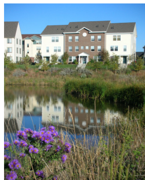
Naturalized Retention Ponds can be used for regional extended detention. Treatment of the WQv upstream is encouraged to maintain better water quality in the permanent pool.
