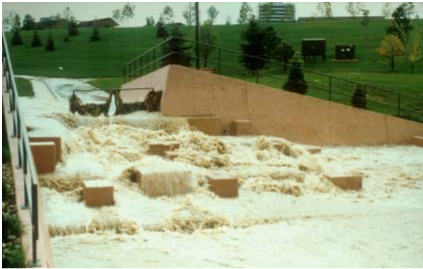
POURED-IN-PLACE CHECK STRUCTURE This is a modified form of a baffle chute structure designed to minimize vertical hazards. Although the structure is appropriate for its setting, the concrete low flow channel and vertical drops of the low flow channel provide no habitat value. The photo on the bottom shows the structure during a minor storm event.
