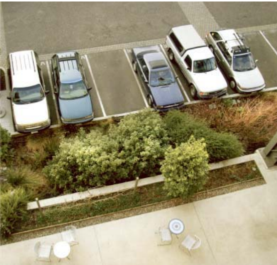
APPROPRIATE PLANTING OF PLD This mix of drought and inundation tolerant plantings requires minimal maintenance. Trees are at the edge of the PLD. Source: City of Portland, Department of Environmental Services
