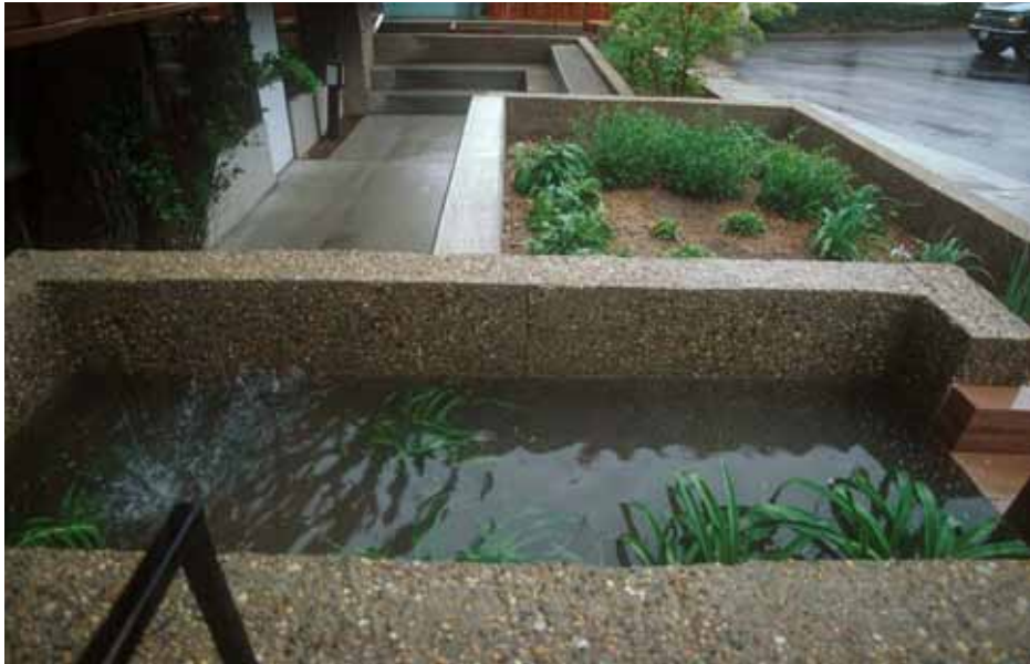
ROOF DRAIN INFILTRATION PLANTER This infiltration planter accepts roof run-off, seen in the foreground, as well as runoff from adjacent parking, in a series of three interconnected infiltration planters. Storm volumes exceeding the capacity of the planters spill into the parking area.
