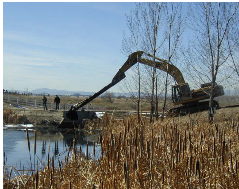
Sediment removal from a forebay.
