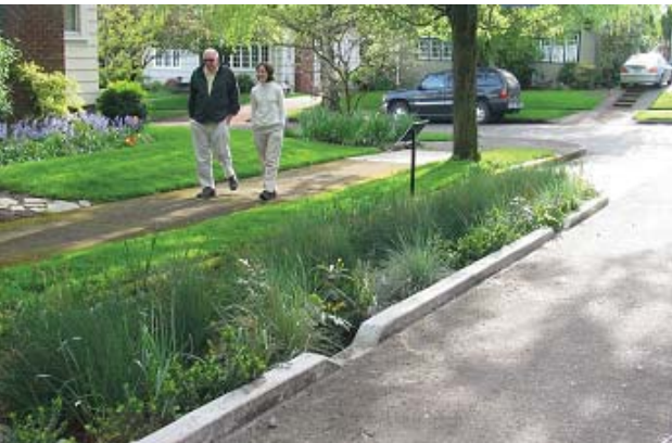
Detail of PLD. Curb cuts divert smaller storm flows to infiltrate into PLD. Larger flows divert to the stormwater system when the PLD fills. Source: City of Portland, Department of Environmental Services
