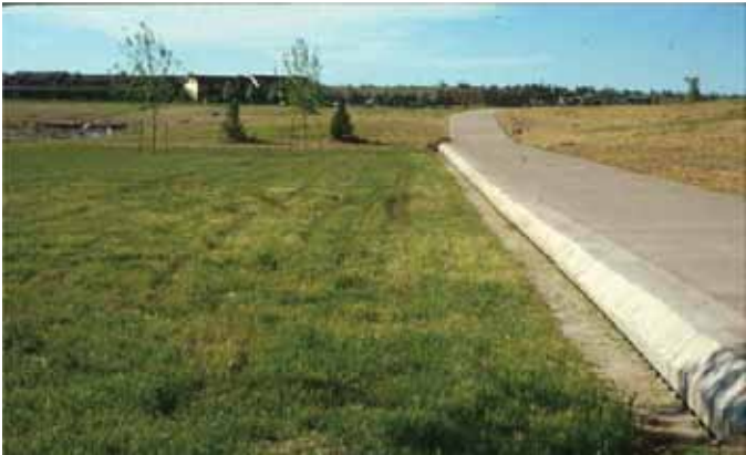
PIPE LEVEL SPREADER A horizontal slotted pipe “level spreader” below the curb evenly distributes storm flows to avoid standing water and disperse concentrated flows.
