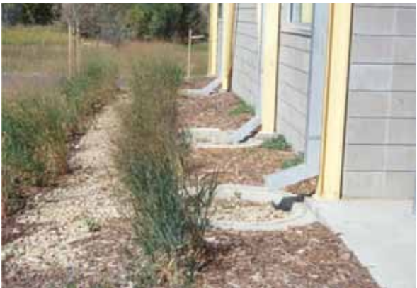
DOWNSPOUT Rooftop runoff from urban housing splashes into rain gardens set in buried concrete pipe adjacent to the building, and then flows on a concrete pan out of the basin.
