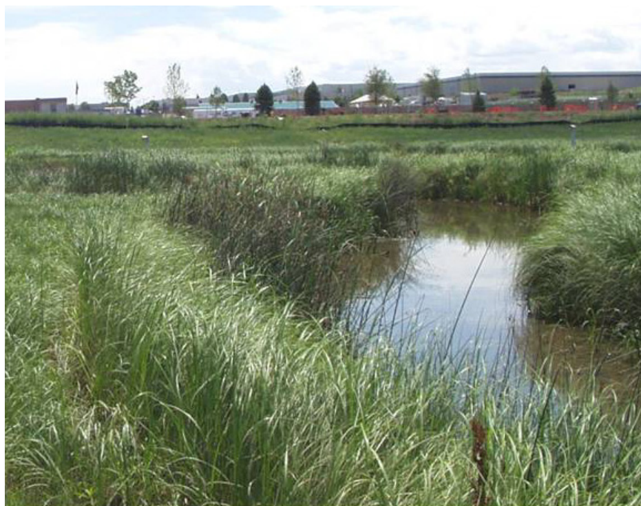
Created wetlands adjacent to the creek provide areas for filtration of stormwater as well as habitat.
