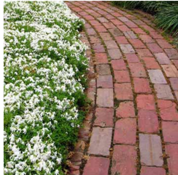
PerVIOUS paving to aid in percolation of runoff water
