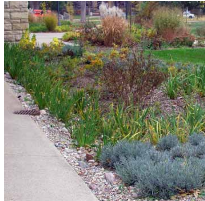
Rain gardens fed from roof runoff that aid in the biofiltering of runoff
