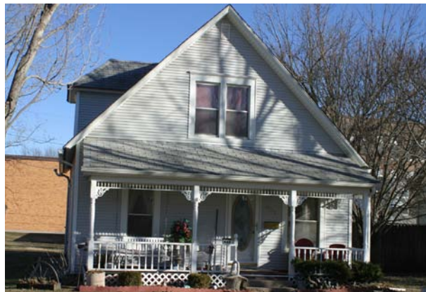
One-and one-half story front gable house in Uptown Ankeny
